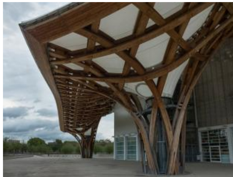
Centre Pompidou Metz
